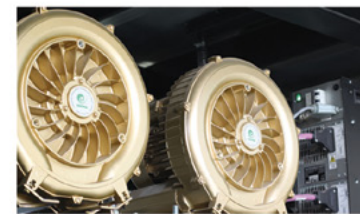
LOCAL Vacuum System
